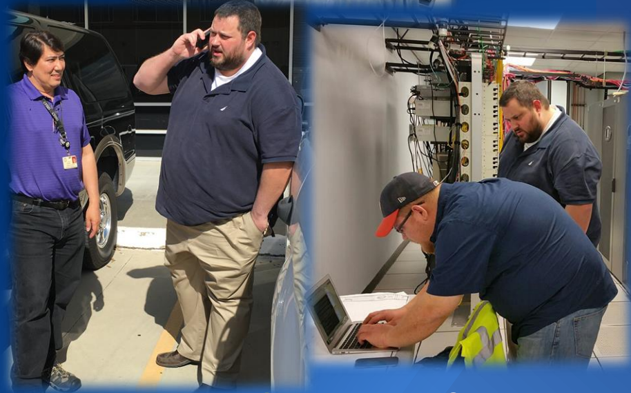
Oscar Villar replacing ASR module.
