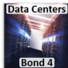
Data Center Upgrades
