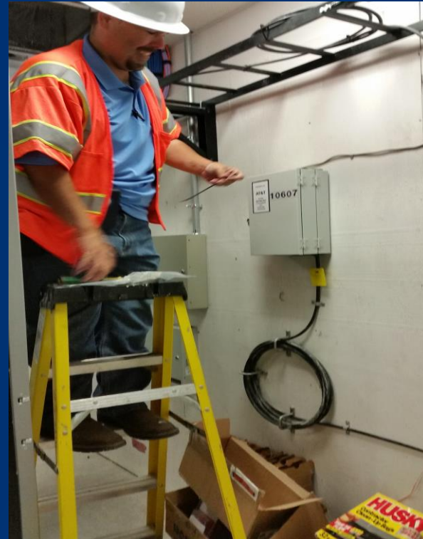
PS/Lightwave technician Pete Cavazos relocating fiber tray
