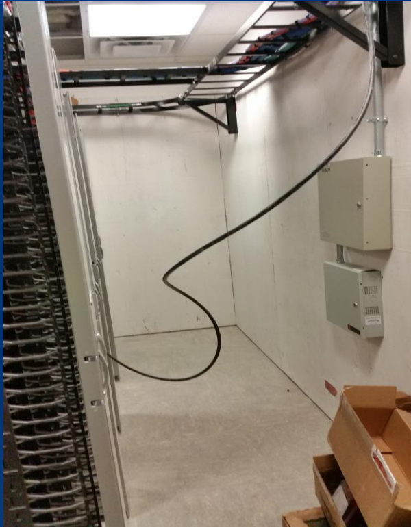
Relocating Lightwave fiber optic cable in MDF.
