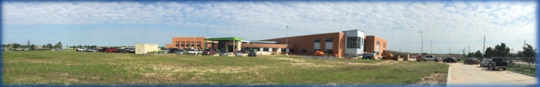
Panoramic View of Woodard Elementary School
