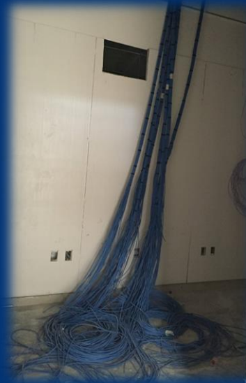
Crews still hard at work pulling cabling for Woodard connectivity.
