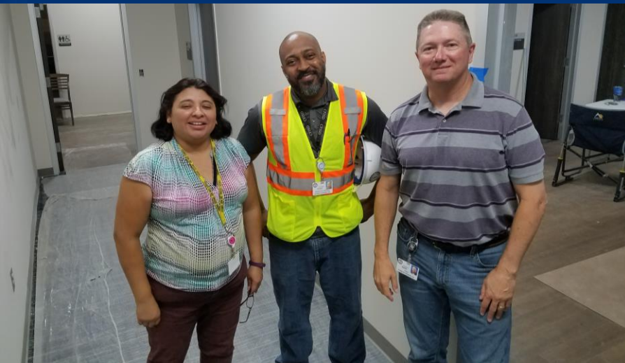
Anna Senties, Tony Rogers, and Bob Rader Working at the New Matzke Installing Network Infrastructure for Connectivity
