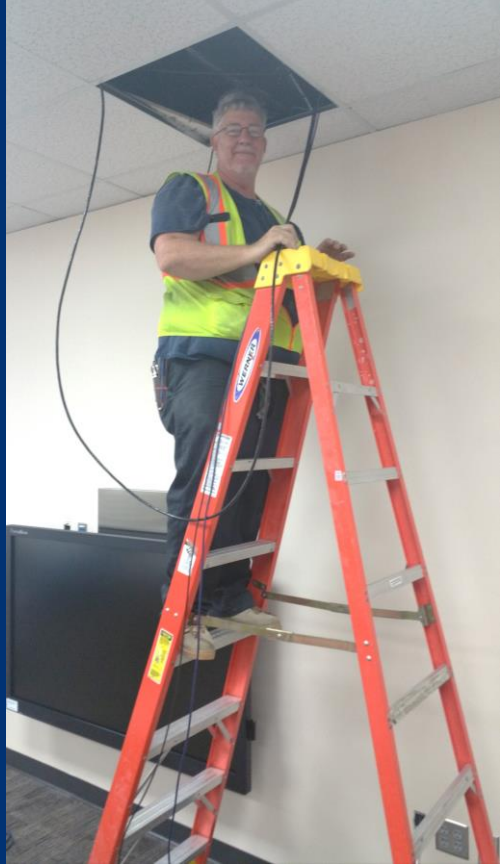
MCA Technicians working at Francone elementary, installing prometean board panels. The installation requires a complex setup with cabling and wall mounting, taking between 30 minutes and 1 hour to complete.
