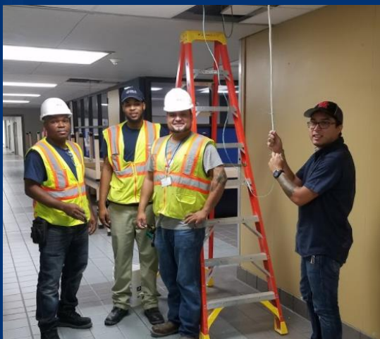
MCA Cabling Team
