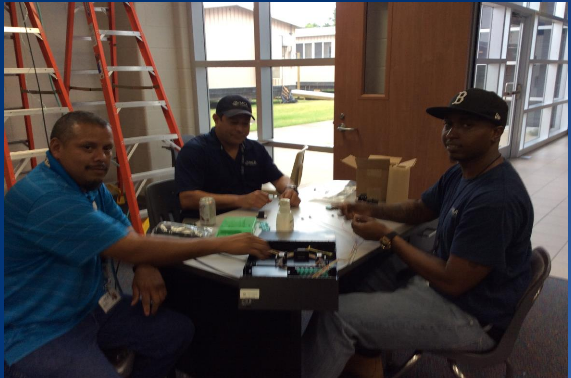
Pictured above MCA terminating the fiber at Spillane MS
